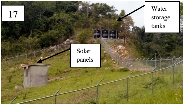
Photo 17 – Solar panels located on top of pump house and black plastic water storage tanks on stand Photo 18 – Two greenhouses alongside the pond
