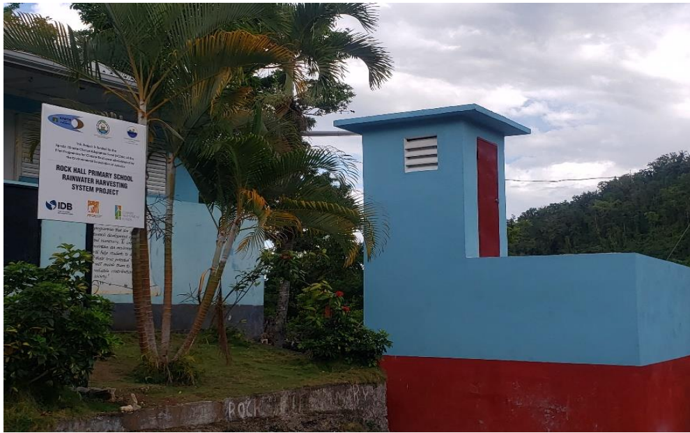
Completed water harvesting tank with pump house (atop)
