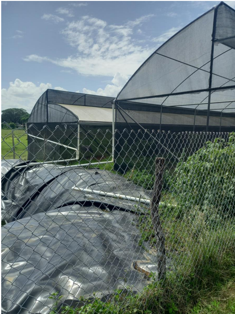
Constructed greenhouses and fenced catchment pond
