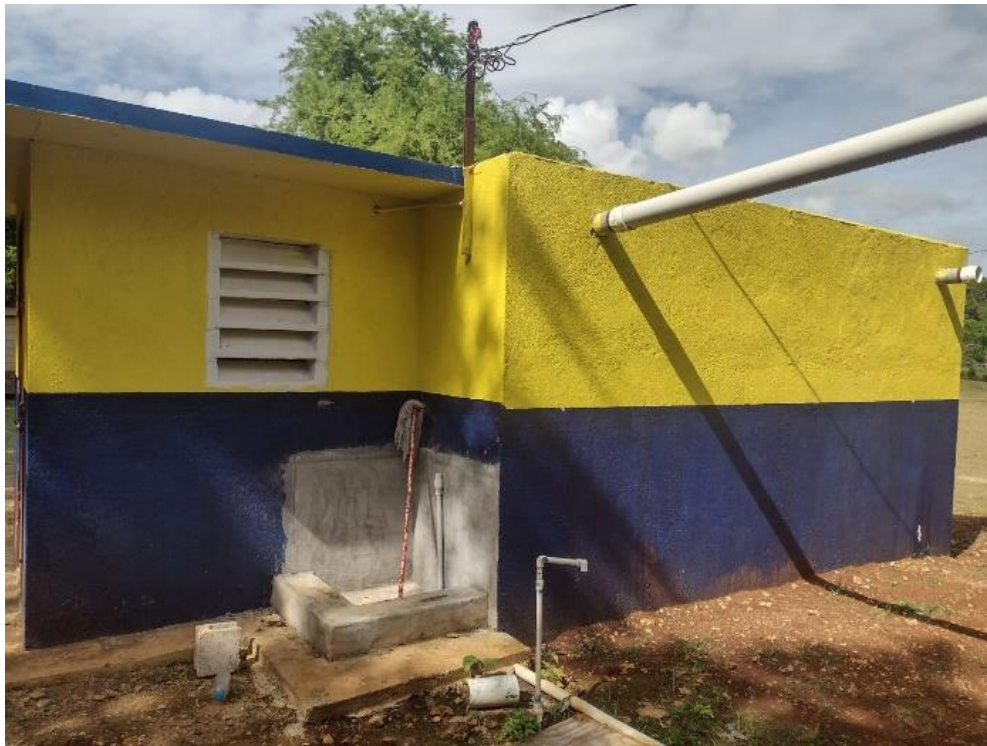
Completed tank with conveyance pipes installed
